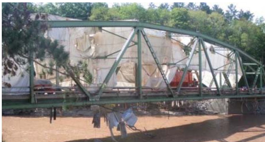
The Prattsville bridge, September 1, 2011. The plastic sheeting is used to contain the sandblasting materials within the construction site, and the bridge was reopened 6 months later by the Department of Transportation, March 19, 2012. This picture copyright © Albany Times Union . 9/2/12, used with permission, courtesy of the Albany Times Union .
