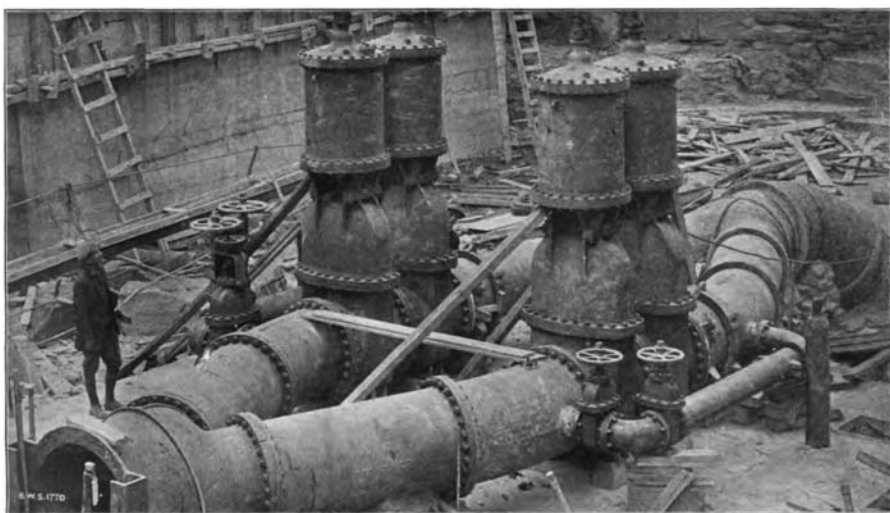
Below: One of the four assemblies of blow-off pipes with hydraulic shut-off valves under the gate-house. Photo courtesy of the Department of Environmental Protection from the Board of Water Supply Annual Report , 1922.
